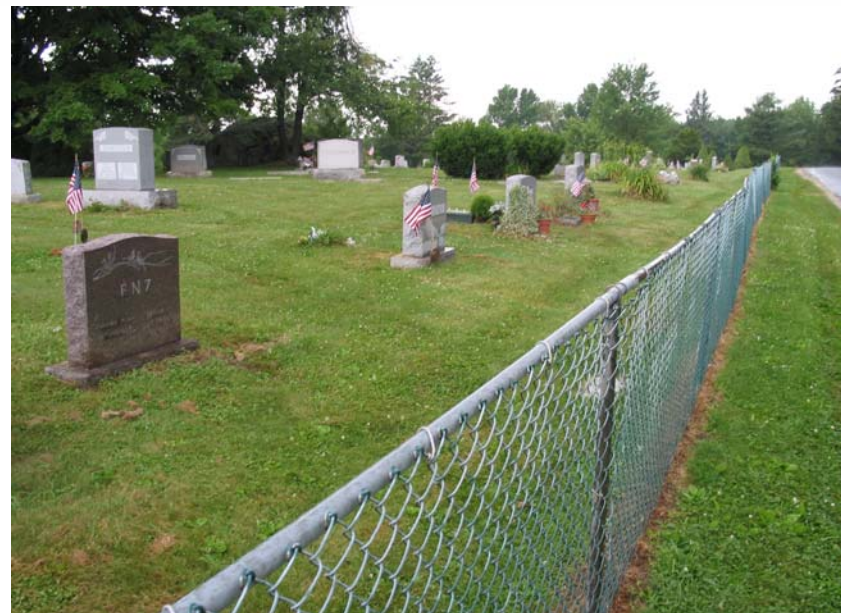
Cemetery fence line looking Northwest along South Road
